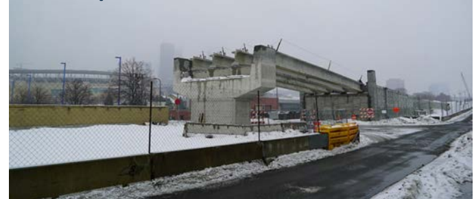
LRT Bridge Pier Construction at Royalston Avenue/North 7 th Street
