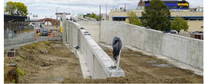
Retaining wall construction at Royalston
